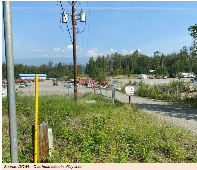
Source: DOWL - Overhead electric utility lines
